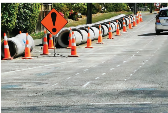
New water pipes ready to install at Huffey and Talbot streets ahead of the major Talbot Street works. PHOTOS: Gavin Oliver
